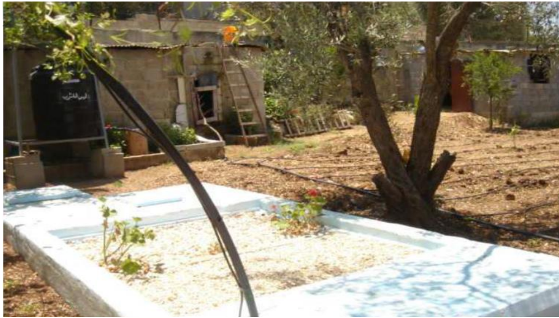
Figure 2-3: Up-Flow gravel filter Grey water treatment technology after construction Source: PHG, 2011
